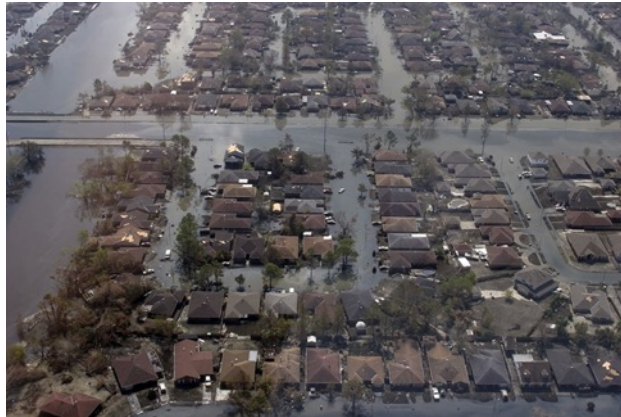
New Orleans flooded and stranded
