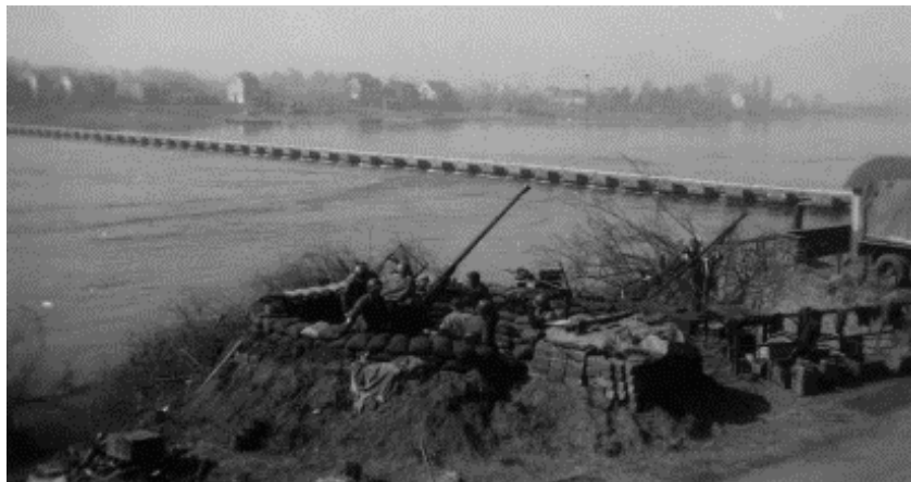
Pontoon Bridge over the Rhine River into Germany
